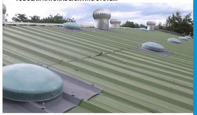
SINGLE BOUNCE DESIGN MAXIMISES VISIBLE LIGHT REFLECTION INSIDE WORK AREA
